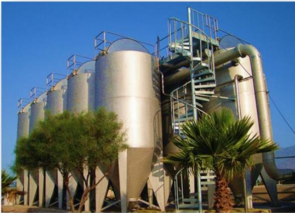
The **DynaLite-Filter** filter employs a backwash rinse that is performed continually while the tank is processing water. An air lift pump, located at the Centre of the module draws the media from the bottom of the filter up into the wash box. As the media is released into the wash box, it falls into the media washer where the filtered solids are separated from the **ZEOSORB**. From there, the filtrate carries the solids out as waste (backwash).
